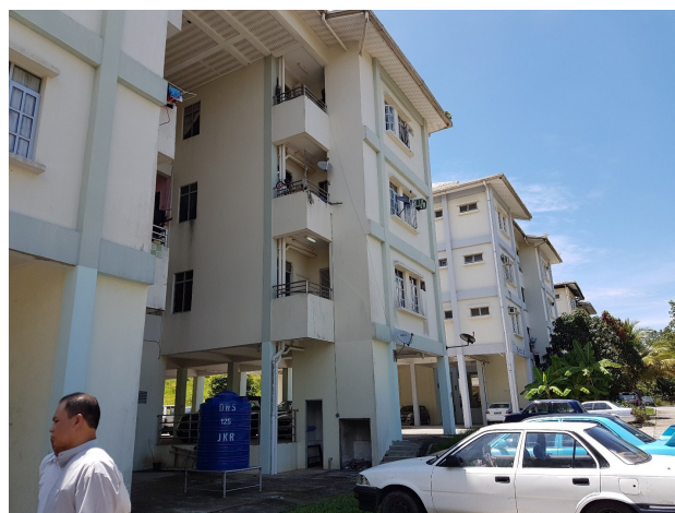
Temporary shelter managed by the Community Development Department (JAPEM)
