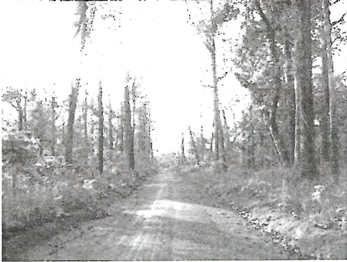
Figure 8 Villages' roads connect from the national road No. 78
