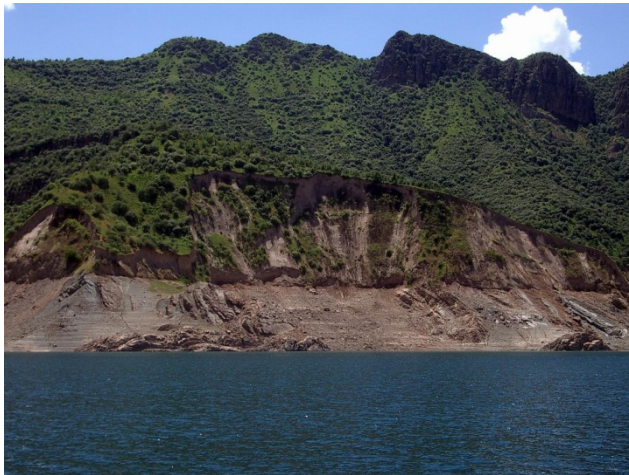
Figure 5-5: Bank Collapse into Nurek Reservoir, Tajikistan
